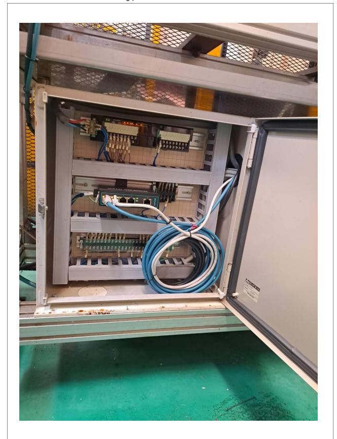
Installation Ethernet-Hub and wiring power SR-X300
